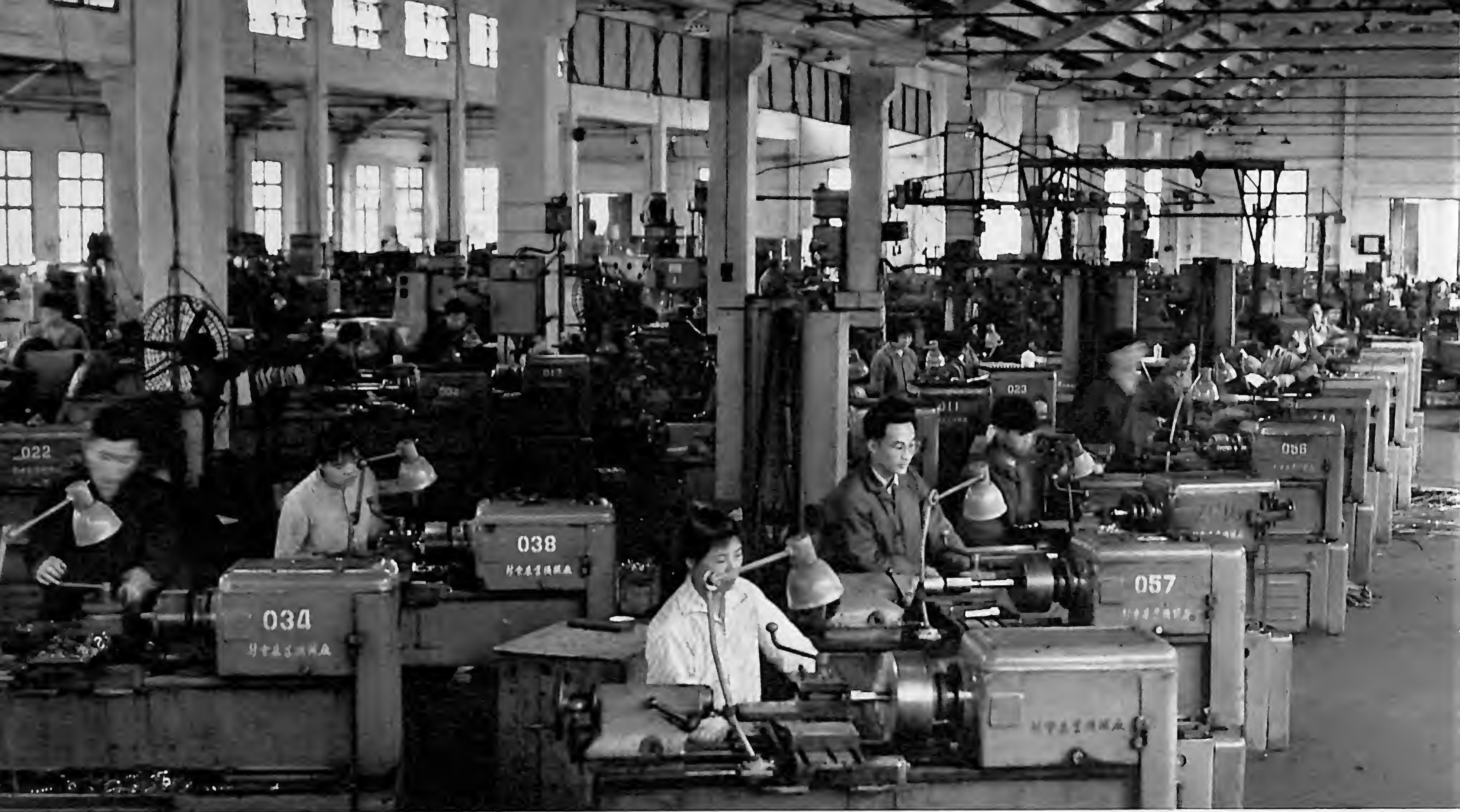
Metal working shop of the farm machinery plant. Its workers designed and manufactured most of the lathes — over 200 of them.
